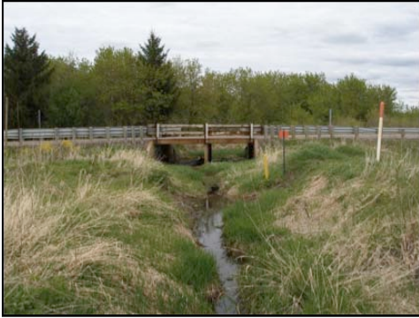
Roadway Bridge - Slovak Valley Creek
